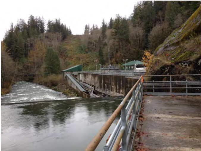
GRD-61.0-N Photo: Adult salmon ladder and water diversion dam for City of Tacoma water supply. Looking W downstream from water intake on river right.
