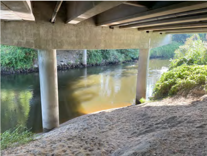
GRD-13.2 Photo: Taken from under Strander Blvd Bridge from the Green River Trail, just upstream from Bicentennial Park.
