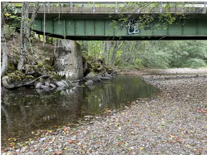
SUNC-0.1 Photo: Looking upstream towards the NF-52 road bridge on Sunday Creek.
