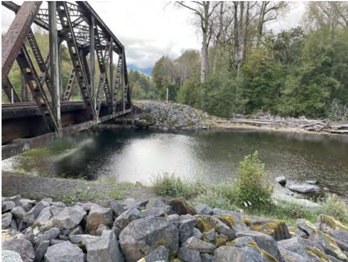
GRD-80.9 Photo: The Green River taken from the BNSF railway bridge at Lester.
