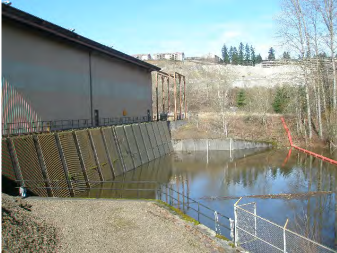
BLAKR-0.3-N Photo: King County Black River Pump Station, from south bank looking north, upstream of pump station. Black River Riparian forest to the right on the photo.
