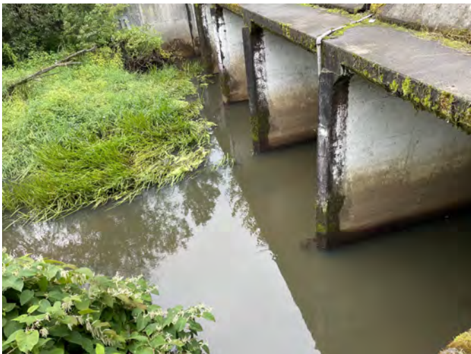
SPBC-1.4 Photo: Springbrook Creek culvert entrance just downstream of SW Grady Way and I-405.
