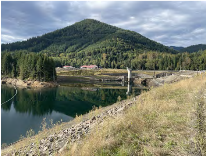
GRD-64.6-N Photo: Howard Hanson Dam looking from the north side of the dam.
