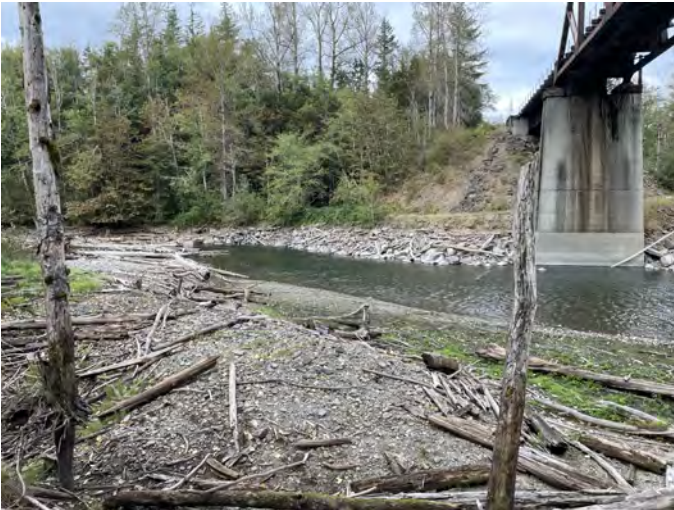
GRD-68.4 Photo: Looking upstream from under the NF-54 bridge just upstream from the Hanson Dam Reservoir.
