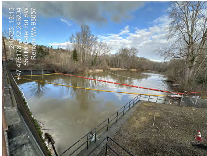
BLAKR-0.4 Photo: Boom placed at King County Black River Pump Station for spill response in February 2025.
