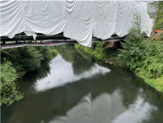
GRD-21.0 Photo: Looking upstream from the pedestrian bridge towards the Meeker Street Bridge (under going renovations)
