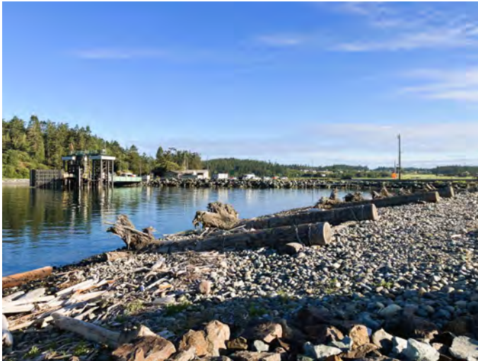
AI-19 Photo: Facing N toward ferry dock and pipe under road to Crockett Lake from boat launch.
