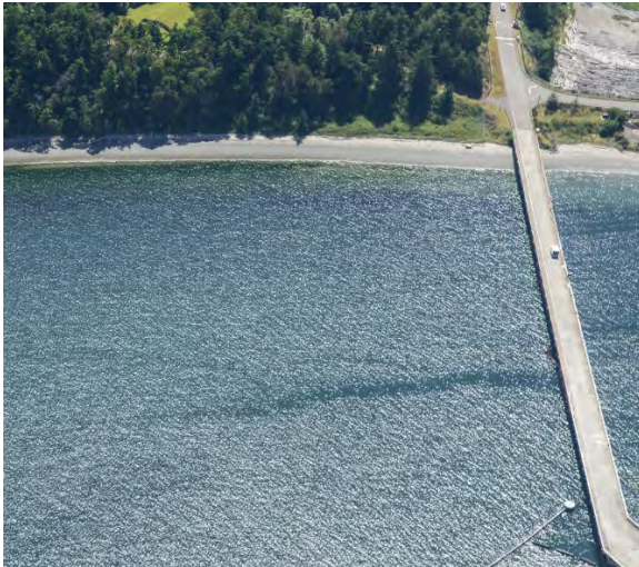
AI-12.3 Photo: Facing E at Navy Region Northwest restricted area and pier on N side of Walan Point.
