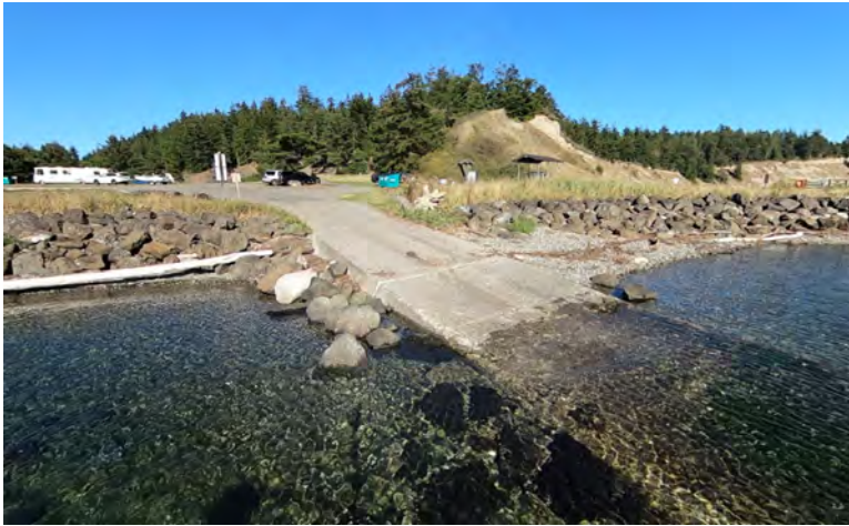
SA-AI-12.1 Photo: Photo taken from onwater toward the west side of the park at the boat launch and camp area.
