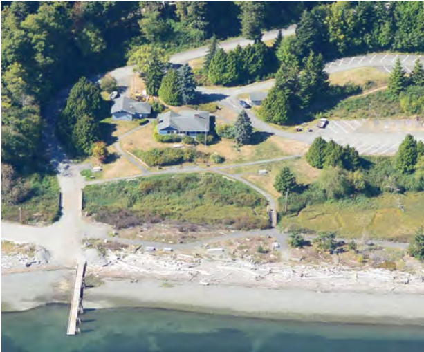
SA-AI-31.2 Photo: Aerial photo (2016), looking toward boat ramp and park from Possession Sound.
