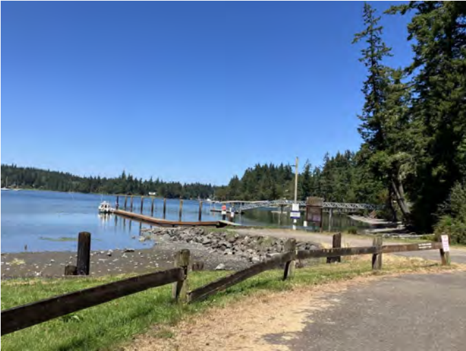
SA-AI-21.1 Photo: Looking NE at ramp and dock into Mats Mats Bay.
