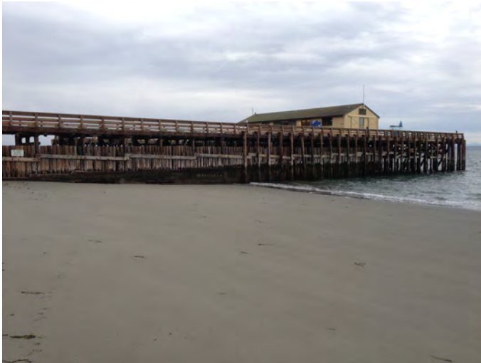
AI-01.1-N Photo: Looking from the beach at the south side of the pier and Science Center.
