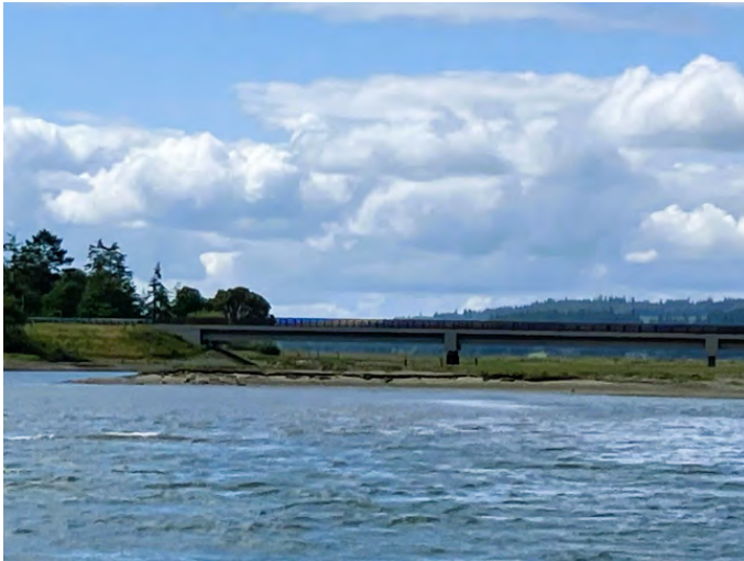
AI-17 Photo: Facing S from inside Scow Bay (Kilisut Harbor) toward fish passage bridge. East is Marrowstone Island, West is Indian Island.
