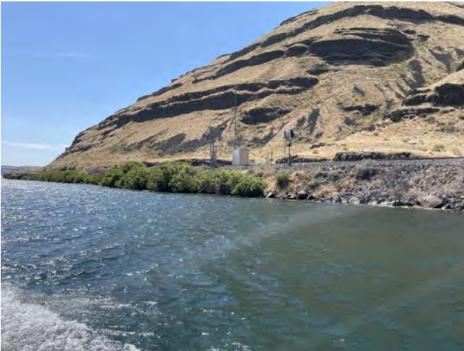
M-308.8R Photo: From boat, looking southwest/downriver towards culvert. Low water conditions (August).
