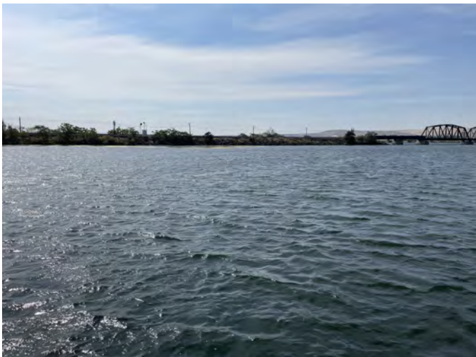
M-323.5M Photo: From riverbank, looking south towards anchor point B and rail bridge. Low water conditions (August).
