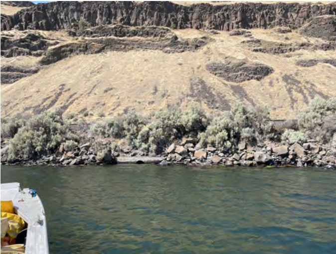
M-304.5R Photo: From boat, looking northwest towards culvert. Low water conditions (August).
