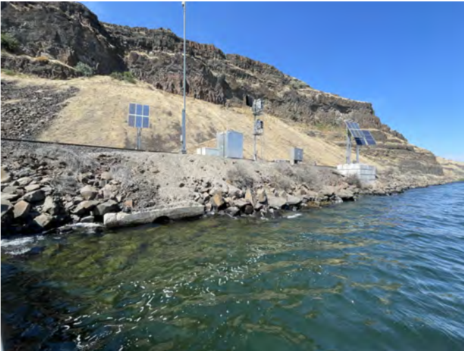
M-303.3R Photo: From boat, looking north towards culvert. Low water conditions (August).
