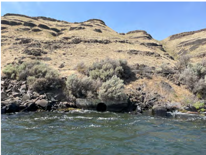
M-310.3R Photo: From boat, looking northwest towards culvert (downriver is to the left). Low water conditions (August).
