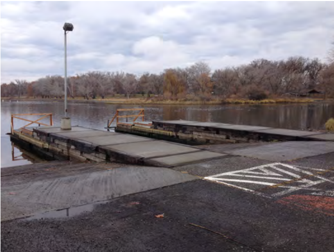
SA-MSN-2.3L Photo: From parking lot, looking east towards ramps and docks with park in the background. River is to the left.
