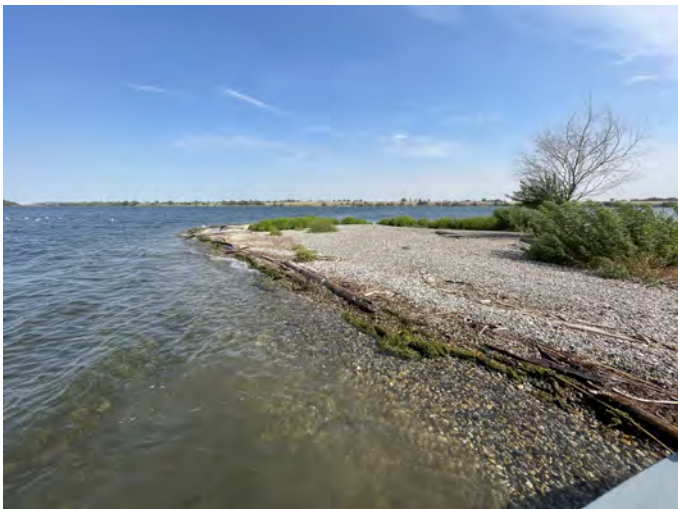
M-322.6M Photo: From island, looking north towards site of deflection boom. Low water conditions (August).
