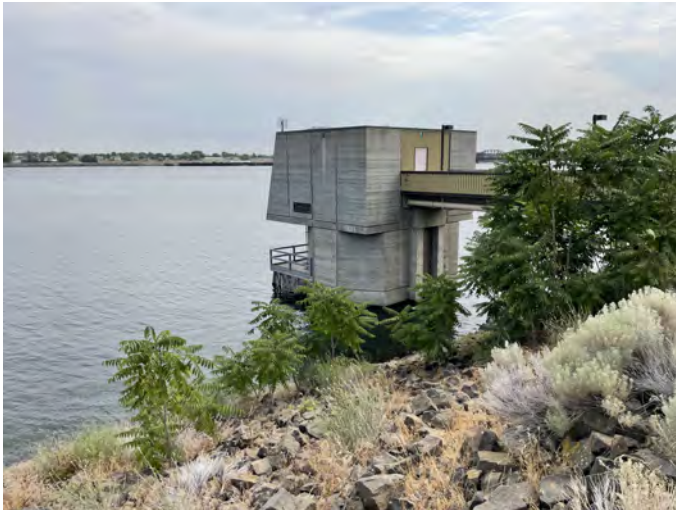
M-328.4R-N Photo: From the riverbank, looking northeast towards the water intake structure.
