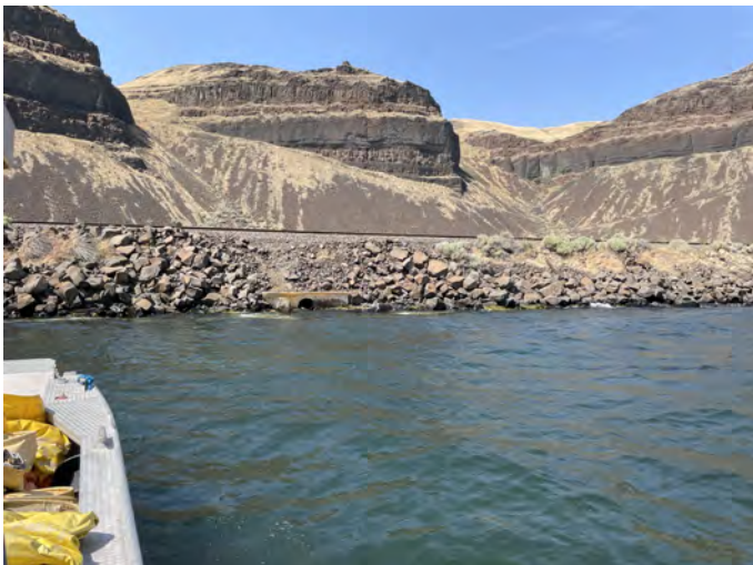
M-311.9R Photo: From boat, looking north towards culvert (downriver is to the left). Low water conditions (August).
