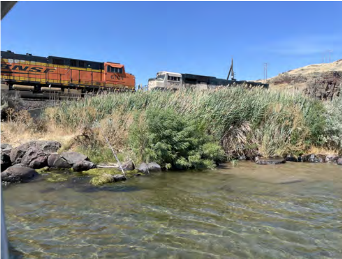
M-302.3R Photo: From boat, looking north towards culvert (obscured by vegetation). Low water conditions (August).
