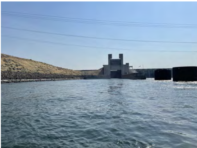
MSN-9.5R Photo: From river, looking east/upriver towards lock. Low water conditions (July).
