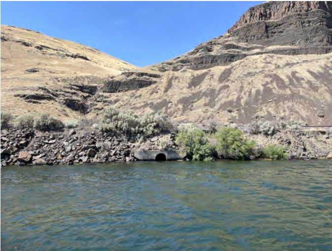
M-306.5R Photo: From boat, looking northwest towards culvert. Low water conditions (August).
