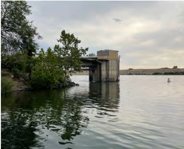
M-340.2R-N Photo: From the boat launch, looking northwest towards the water intake structure.
