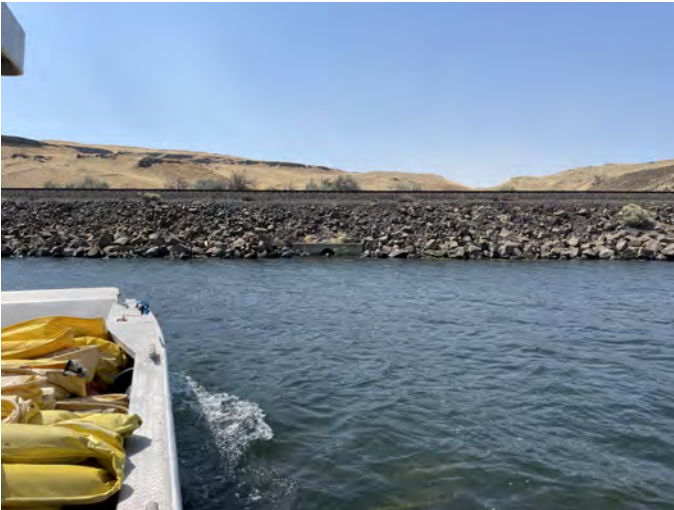
M-314.6R Photo: From boat, looking west towards culvert (downriver is to the left). Low water conditions (August).
