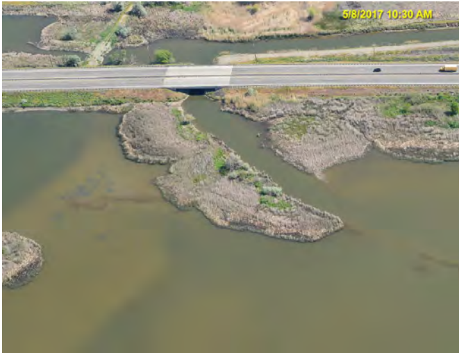
M-320.7L Photo: From above the pond, looking northeast towards highway bridge. High water conditions.
