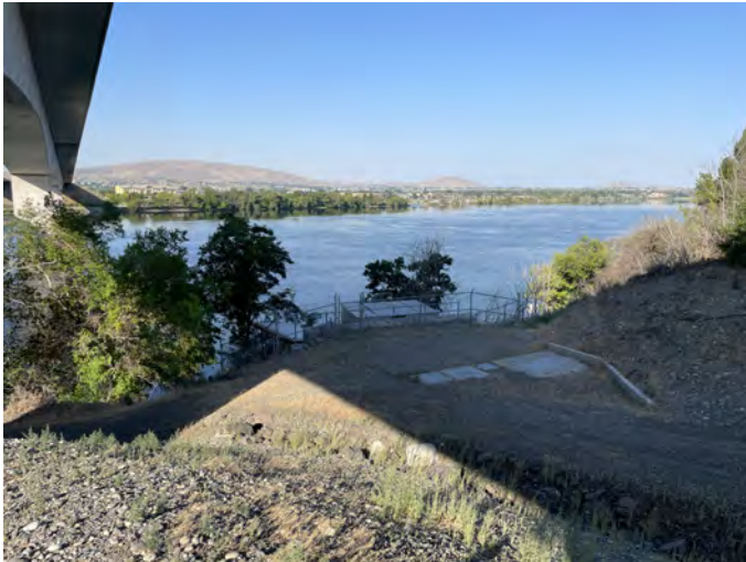
M-336.1L-N Photo: From W Court St, looking southwest towards the water intake structure.
