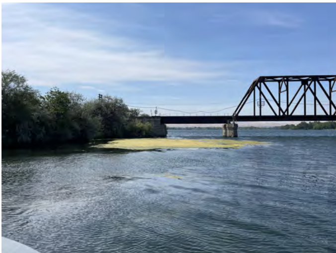
MSN-1.5L Photo: From boat, looking southwest towards anchor point B at bridge. Low water conditions (July).
