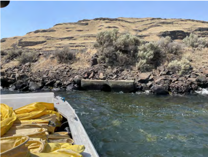
M-310.8R Photo: From boat, looking northwest towards culvert (downriver is to the left). Low water conditions (August).
