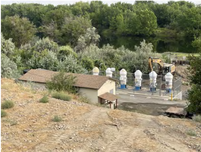
YAK-3.5R-N Photo: From the canal, looking north towards the water intake structure.
