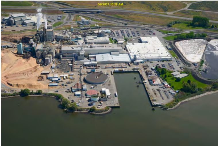
M-316.5-N Photo: From above the river, looking east towards the facility. Photo taken in May 2017.
