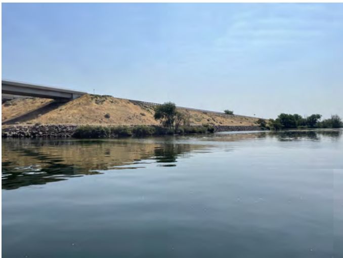
MSN-2.1L Photo: From boat, looking east towards anchor point A (highway 12 bridge in background). Low water conditions (July).
