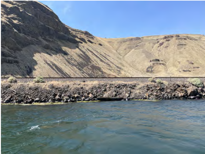
M-309.8R Photo: From boat, looking west towards culvert (downriver is to the left). Low water conditions (August).
