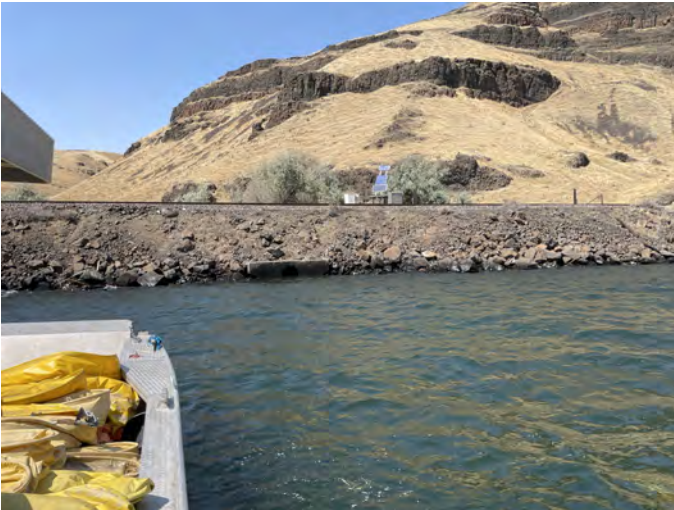
M-311.4R Photo: From boat, looking north towards culvert (downriver is to the left). Low water conditions (August).
