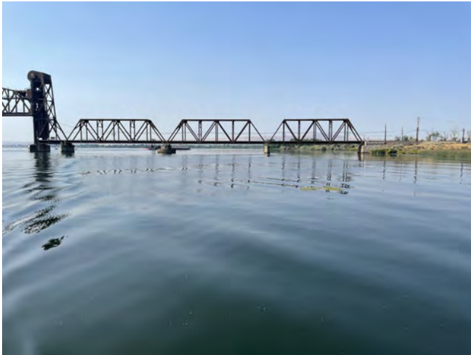
MSN-1.5R Photo: From river, looking southwest towards bridge. Low water conditions (July).
