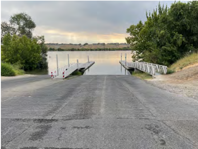
SA-M-340.1R Photo: From parking lot, looking east towards river. Downriver is to the right.
