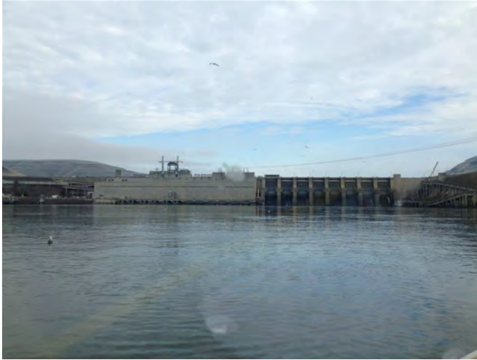
SLOMO-41.4-N Photo: View of the Lower Monumental Lock and Dam from down river in the Snake Ice Harbor Pool
