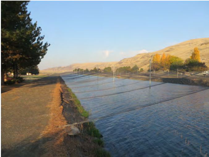
SLOMO-58.3R-N Photo: View of one of the fish rearing tanks, looking west.
