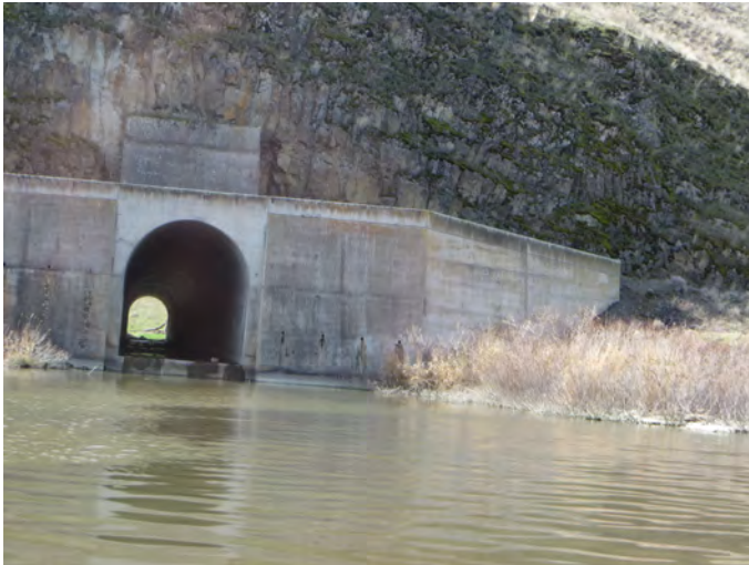
SLOMO-56.0L Photo: From inside inlet, looking at entrance to large culvert.
