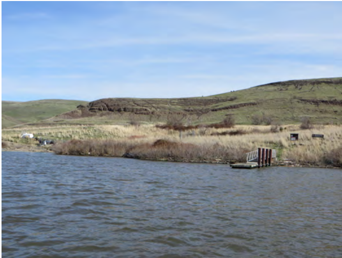
SLOMO-47.7R-N Photo: From near Skookum HMU boat dock, looking downstream at water intake pumps and shoreline habitat.
