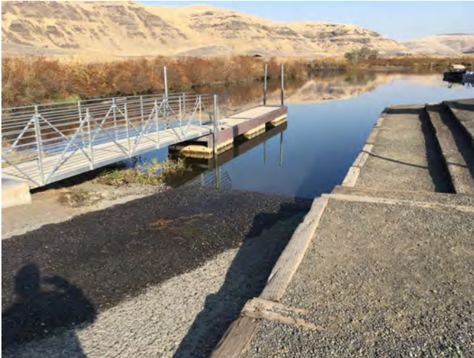
SA-SLOMO-66.0L Photo: From top of Texas Rapids boat launch, looking out towards the exit of the boat basin.
