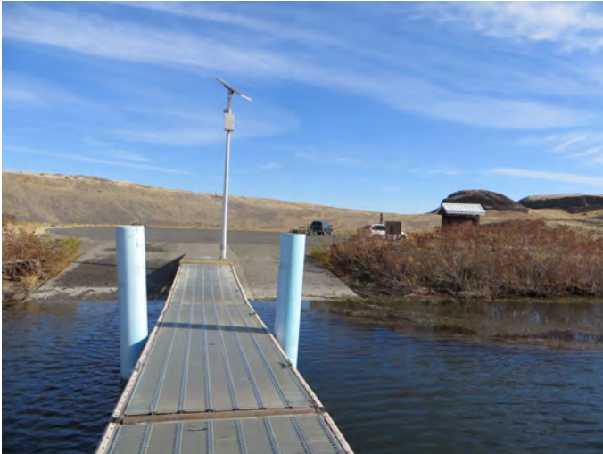
SA-SLOMO-51.0L Photo: From the end of the boat dock, looking northeast at the boat ramps and parking lot of Ayers Boat Basin.
