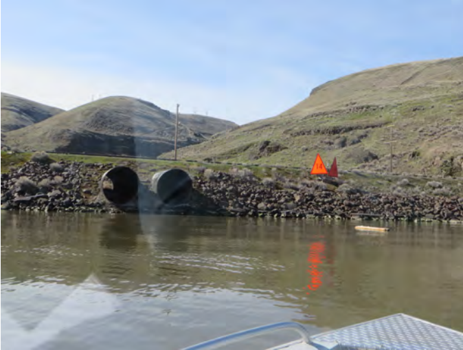
SLOMO-48.4L Photo: From river looking southeast at culverts at river marker 14.
