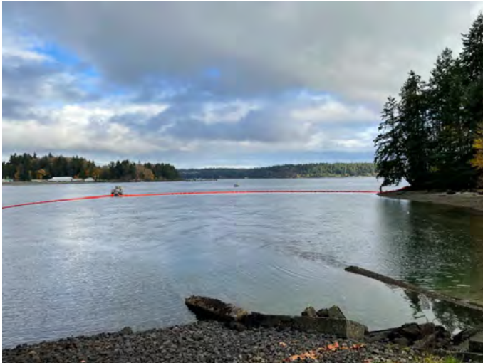
CPS-92 Photo: From near anchor point A, looking northeast with workboat at apex of chevron. Photo taken at drill in November 2023.
