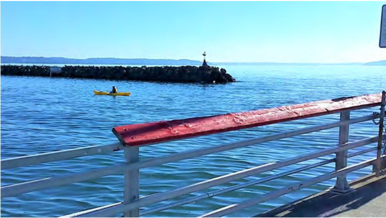
CPS-111 Photo: From A at base of pier near bathrooms, looking southwest across marina inlet to edge of rock jetty. Taken at high tide, +11ft.
