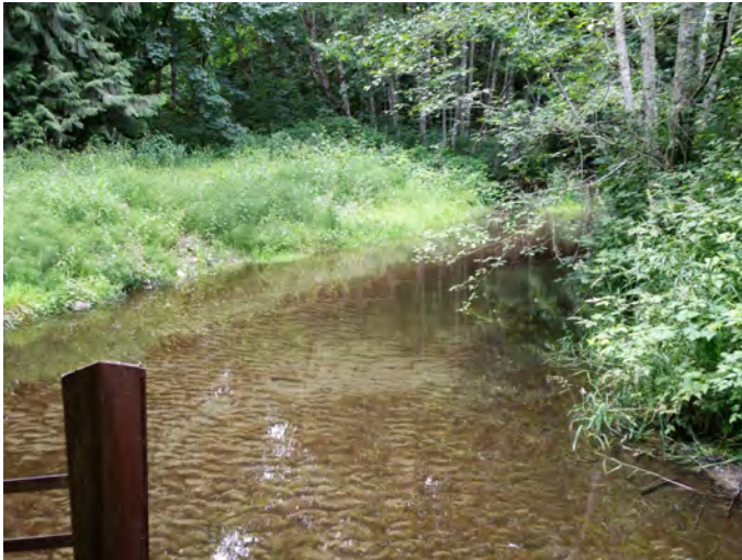
CPS-70-N Photo: Freshwater intake structure on Gorst Creek that feeds hatchery.
