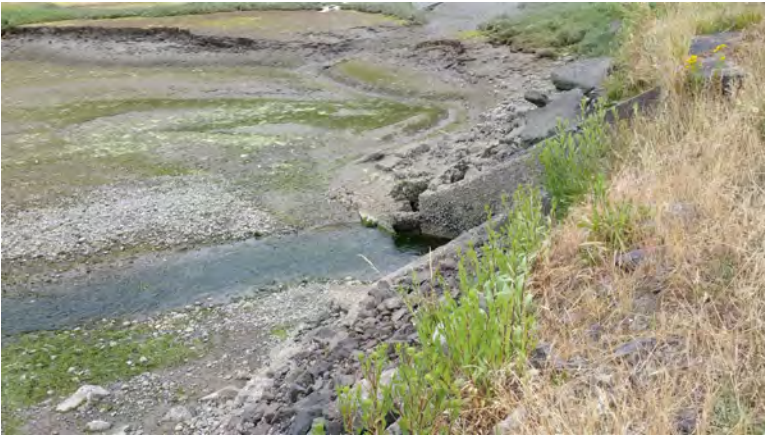
CPS-73e Photo: Looking N at culvert from roadway at +5ft tide.
