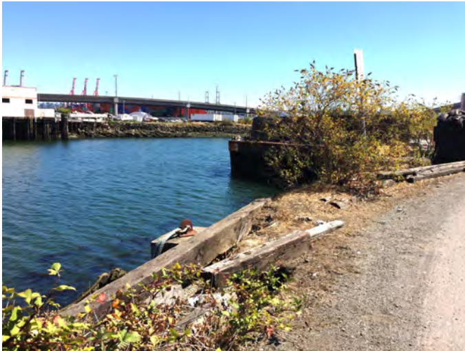
DWW-0.8 Photo: From Chelan Ave NW at barge tie-up (anchor A), looking SE at barge and across Duwamish at Harbor Island. Terminal 12 park is hidden behind barge.
