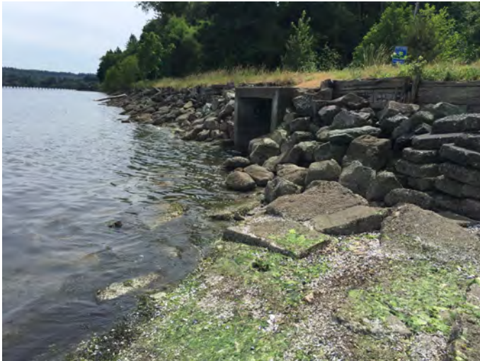
VI-2e Photo: On beach, east of road, looking S at entrance to culvert. Taken at +8ft tide.
