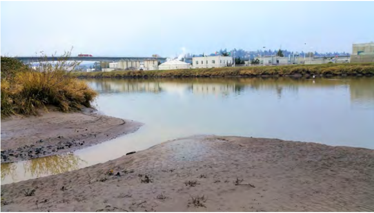
PYLPR-1.6 Photo: On Puyallup River right, looking southeast across levee breach into wetland area. Taken at +6 ft tide, 2400 cfs, 11.6 ft height.
