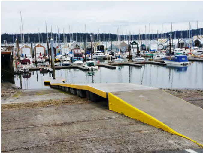
SA-CPS-21 Photo: From top of boat ramps, looking East at marina and Port Orchard.
