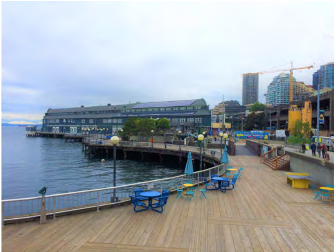
CPS-32-N Photo: From Waterfront Park, looking NW at Aquarium and small water intake building.
