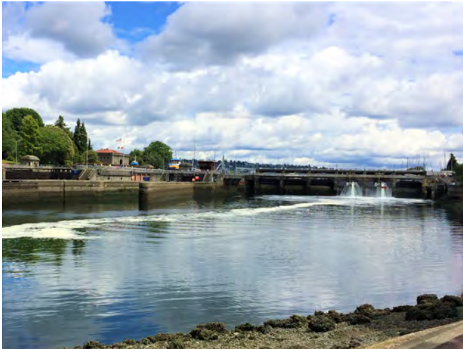
CPS-30-N Photo: From downstream at Commodore Park, looking east at Ballard Locks, spillway and fish ladder.
