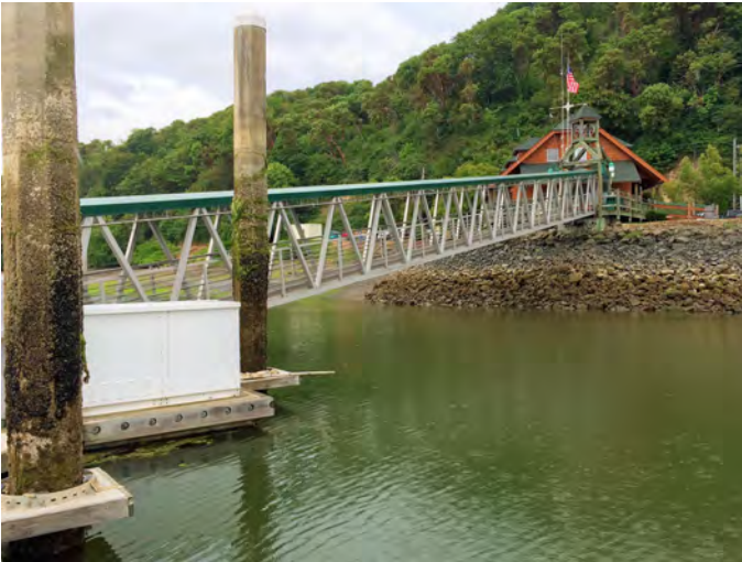
CPS-132a Photo: From dock, looking N at marina parking lot. Taken at -1 ft (low) tide.
