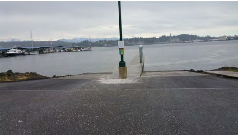
SA-CPS-70 Photo: Looking NW down boat ramp
