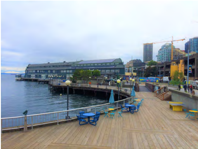
CPS-40 Photo: From Waterfront Park, looking N at aquarium. Intake building at far left.
