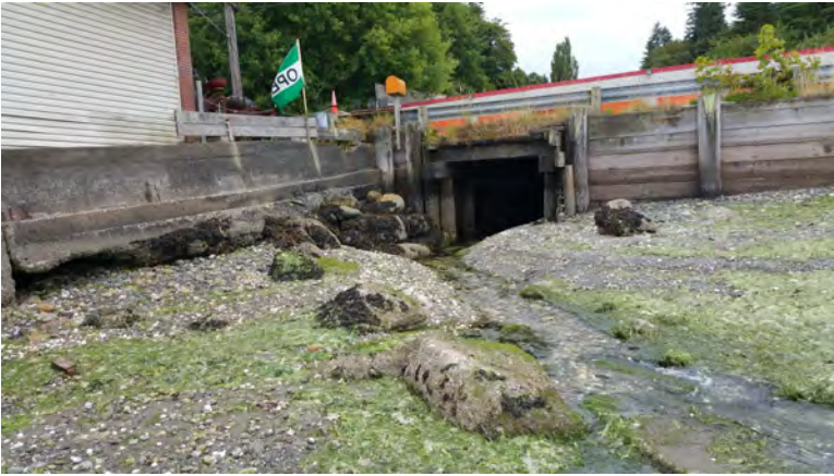
CPS-75e Photo: Looking S toward culvert entrance at +6ft tide.
