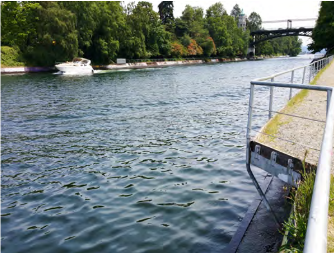
CPS-30 Photo: From south side of Cut at A, looking NW towards UW and collection point (white sign) at anchor point B. Note water-level ledge in foreground.
