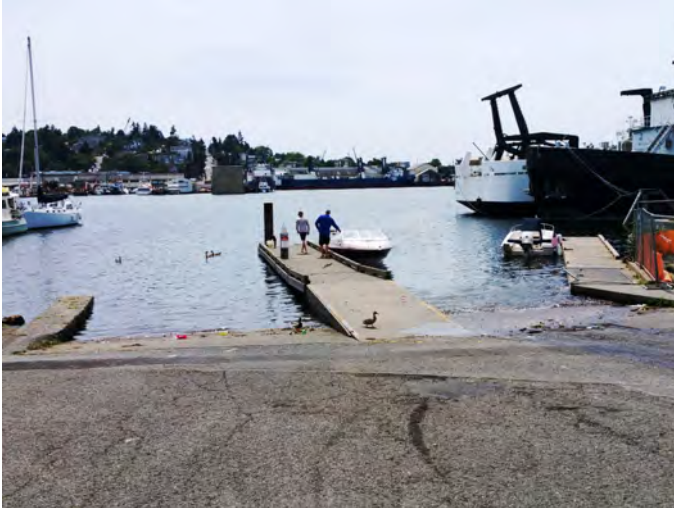
SA-CPS-31 Photo: From top of ramps looking S at shipping canal.
