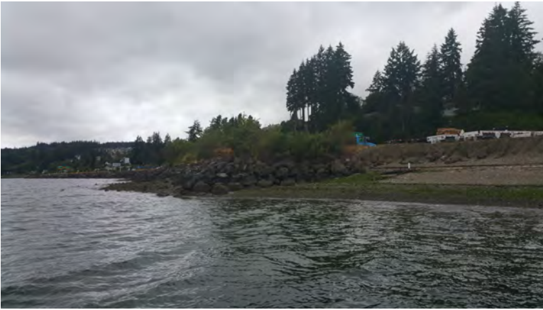
CPS-84 Photo: Looking NW toward anchor point A and collection point.
