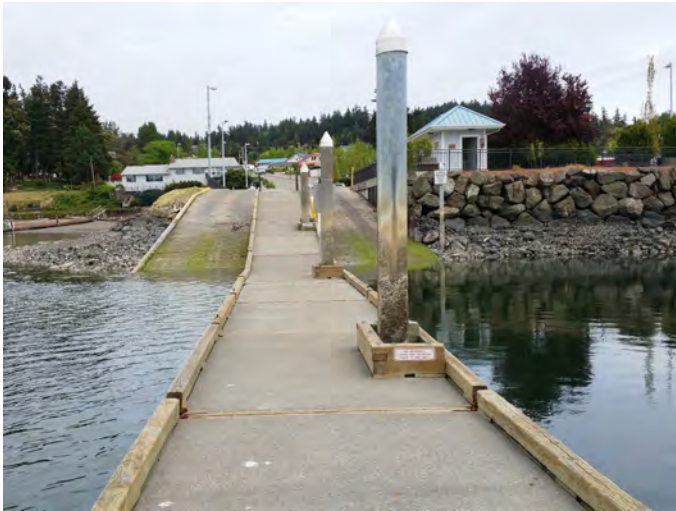
SA-CPS-10 Photo: From the dock, looking N at the twin ramps and elevated parking area with restroom.
