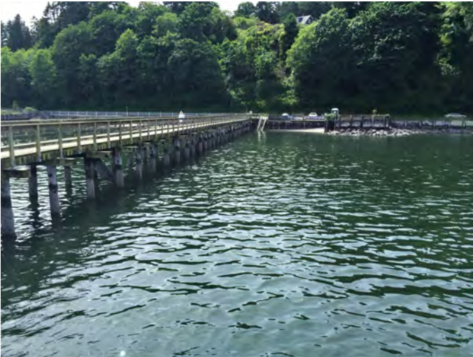
VI-3 Photo: From end of dock, looking SW at parking area and ladder. Taken at +8ft tide.
