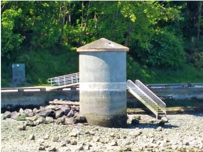
CPS-170-N Photo: Point Defiance pump house intake structure as seen from the water at low tide.
