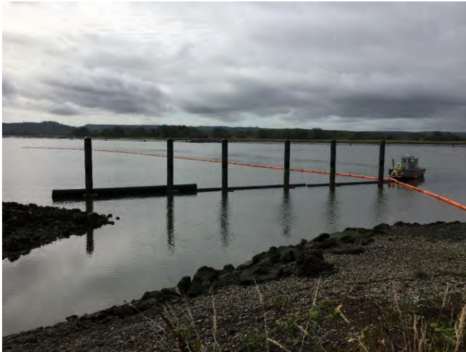
GH-5 Photo: From boat ramp, looking southeast during a deployment drill with Rennie Island in the background. Photo was taken in fall 2017.
