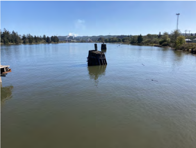
CHER-2.2L Photo: From dock, looking southeast/upriver. Photo was taken in early October.
