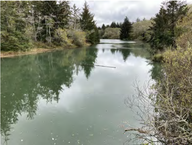
JESS-0.4L Photo: From southeast corner of bridge, looking south/downstream. Photo was taken in early October.
