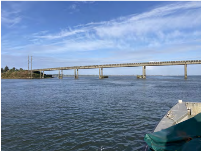
GH-12 Photo: From Elk River, looking northwest towards western end of bridge. Photo was taken in early October.
