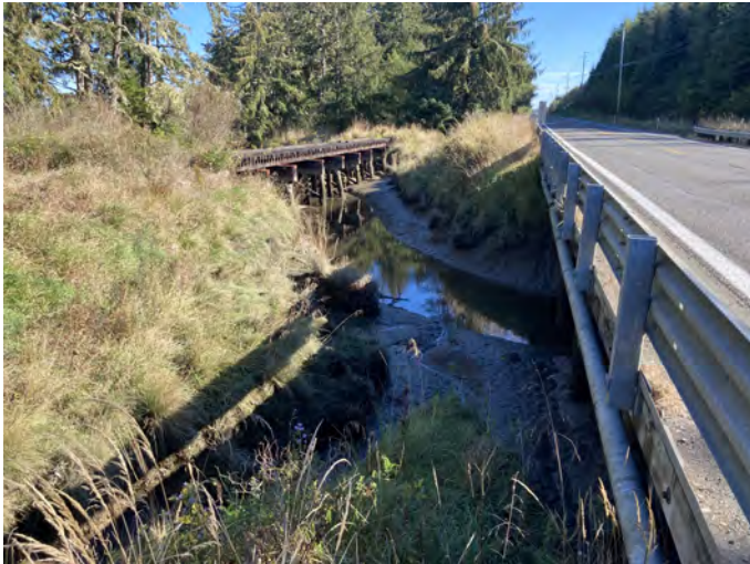
INDC-0.1 Photo: From left bank of creek, looking northeast/downstream towards rail bridge. Photo was taken in early October.
