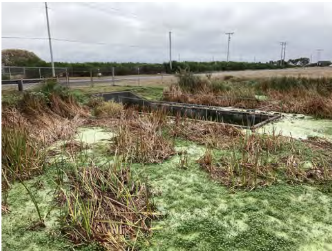
GH-1 Photo: From dock on canal, looking southeast towards culvert. Photo was taken in early October.
