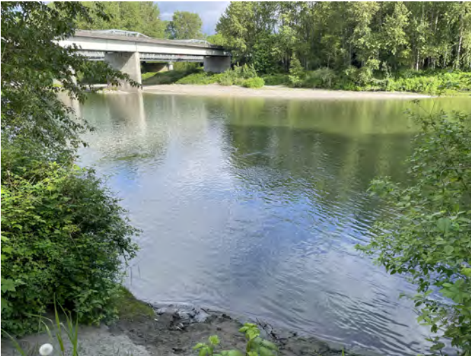
STLGR-11.1 Photo: Stillaguamish River just upstream of the I-5 bridges in Arlington looking north.
