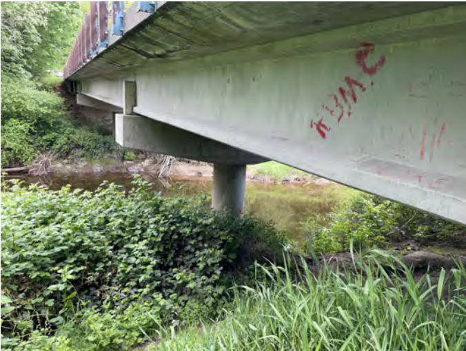
PILC-0.1 Photo: Pilchuck Creek from under 236th St NE bridge.
