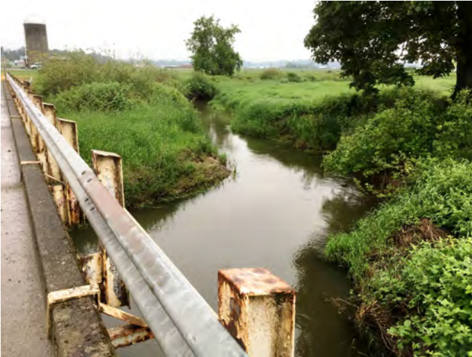
SUMR-12.2 Photo: On Sumas River right, looking NW downstream at strategy location. Taken 5/31/17.
