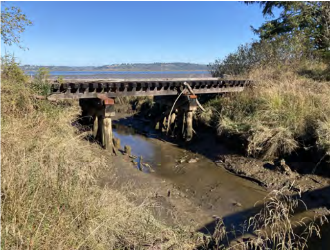
CHPC-0.1 Photo: From left bank of creek, looking north across the harbor. Photo was taken in early October.
