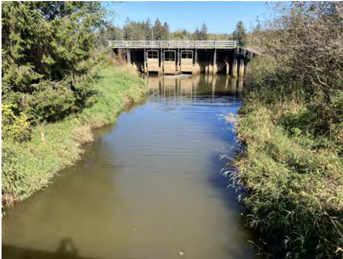
CHER-2.5-N Photo: From First Street bridge over Mill Creek, looking northeast towards the gate. Photo was taken in October.
