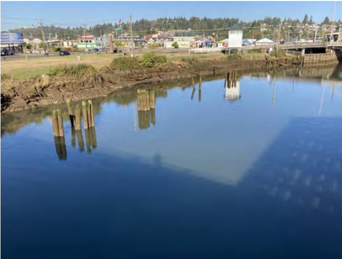
WSHR-0.2R Photo: From the Heron Street Bridge, looking northwest towards anchor point A at the park. Photo was taken in early October.
