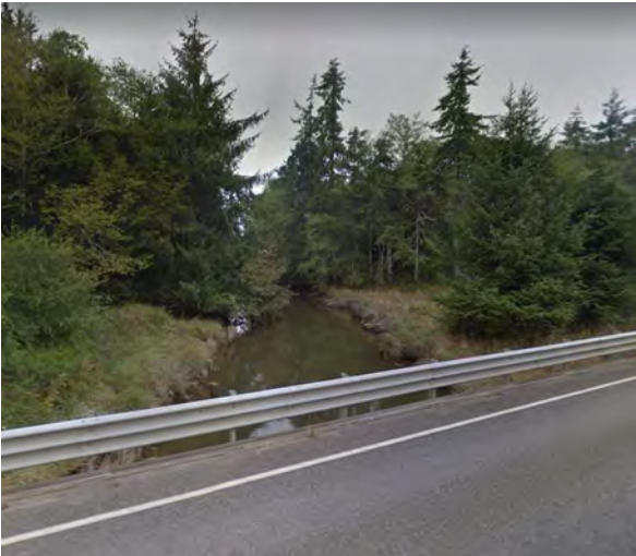
OLRC-0.2 Photo: From middle of WA-105 bridge, looking north/downstream. Photo was taken in August.
