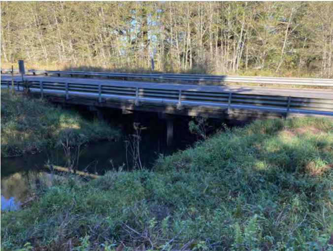
CMBC-0.1 Photo: From right bank of creek, looking northwest/downstream towards bridge. Photo was taken in early October.
