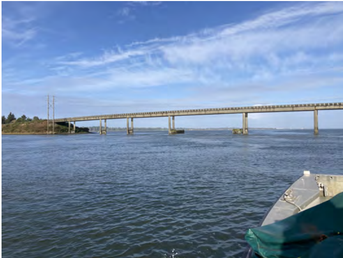
GH-11 Photo: From Elk River, looking northwest towards western end of bridge. Photo was taken in late October.
