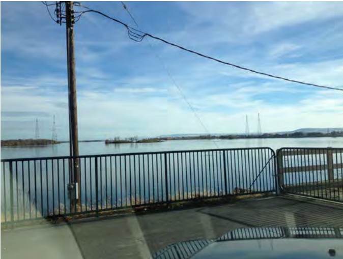
M-326.1M Photo: M-326.1M View of Indian Island from upstream water intake facility.
