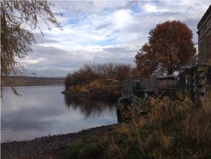
MSN-4.5L Photo: Picture of water intake.
