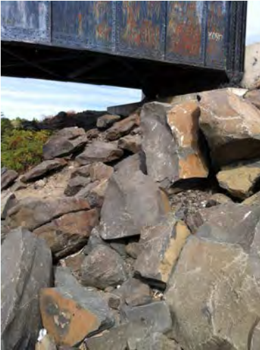
M-323.4M Photo: Northern anchor area
