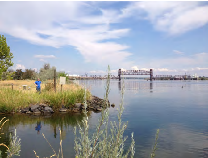
MSN-1.0R Photo: From basin entrance, looking northeast/upriver towards US-12 bridge.
