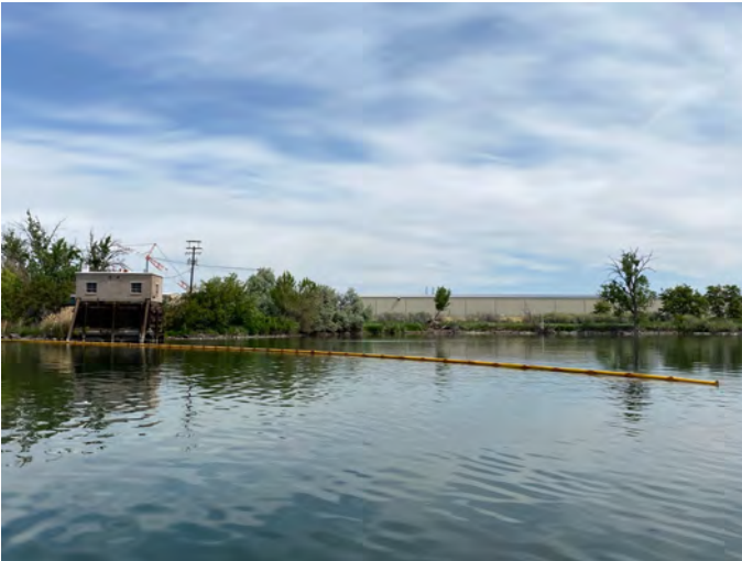
M-326.5L Photo: Facing NE looking at boom protecting water intake facility
