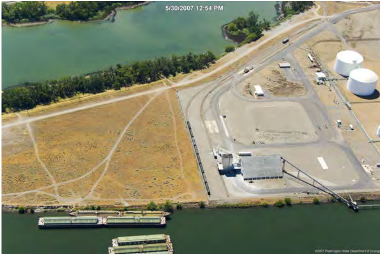
M-323.2R Photo: Aerial overview of collection area.
