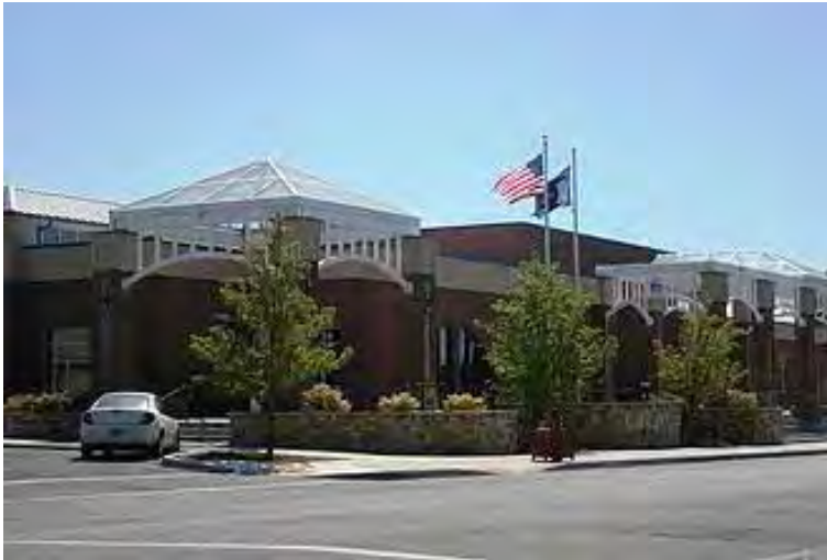
M-293.0L-N Photo: City of Umatilla Public Works Department
