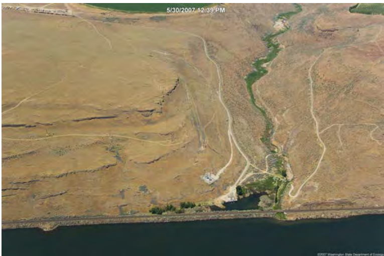
M-302.3R Photo: Aerial view of pump house, creek & train bridge
