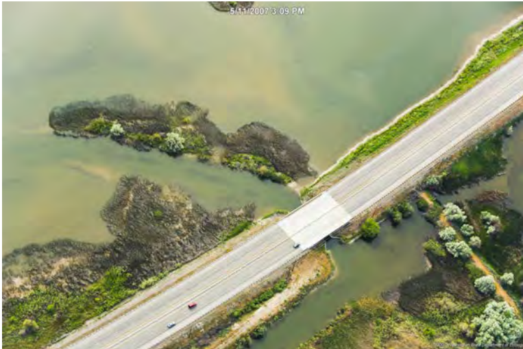
M-320.7L Photo: Highway 12 crossing Casey Pond.
