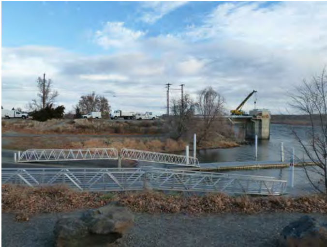
M-340.2-N Photo: View of the Richland City water intake facility (agricultural) from the boat launch to the south
