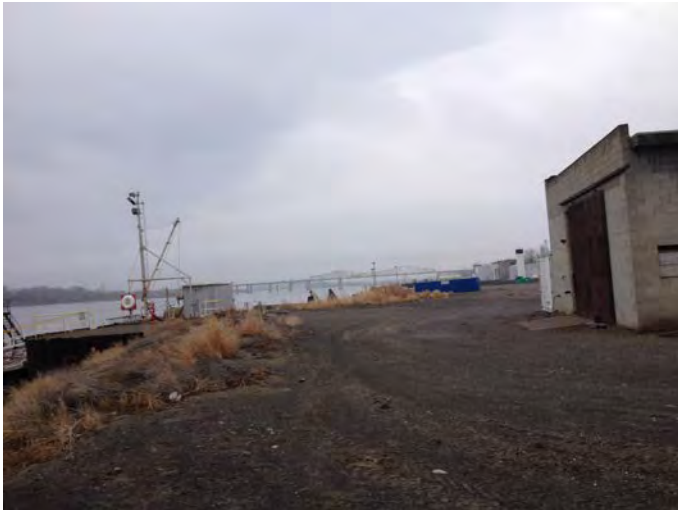
MSN-2.8-N Photo: Tidewater Pasco Facility Boom Storage Locker
