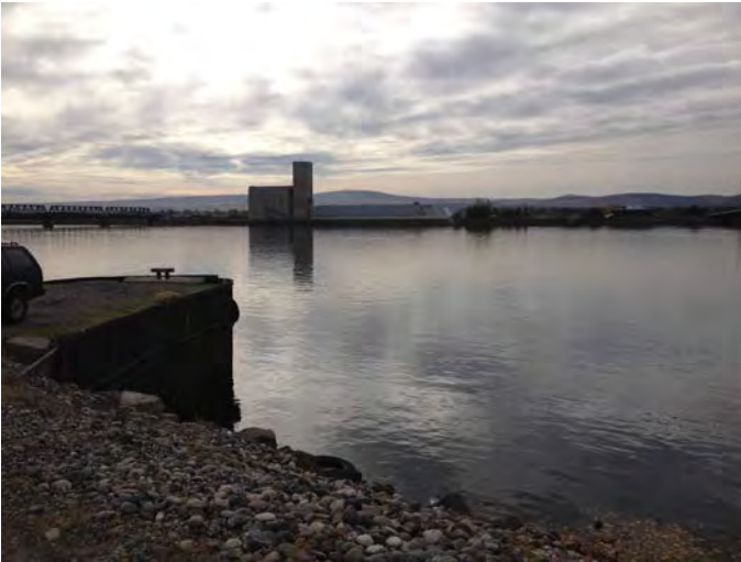
M-328.4L Photo: View of shoreside anchoring position
