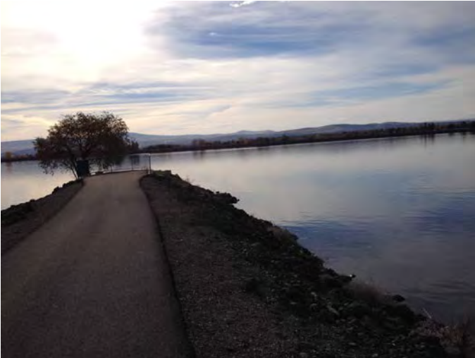
M-327.1L Photo: Looking down the pier at the collection area.
