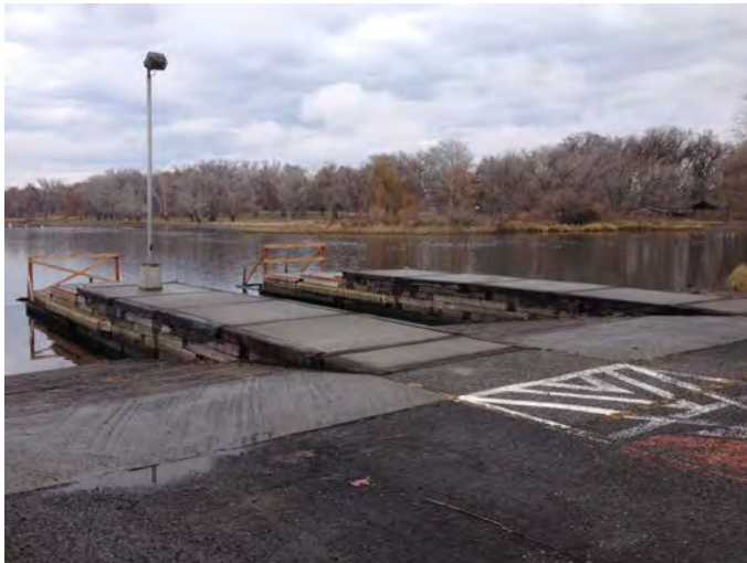
SA-MSN-2.3L Photo: Hood Park USACE boat launch
