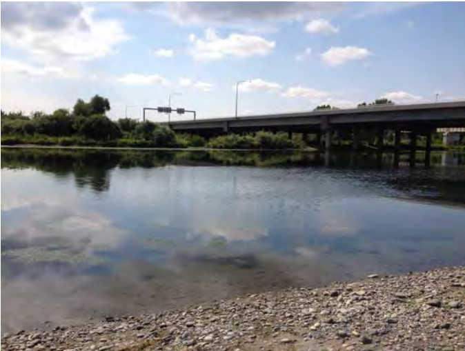
YAK-2.1L Photo: View of collection point facing bridges
