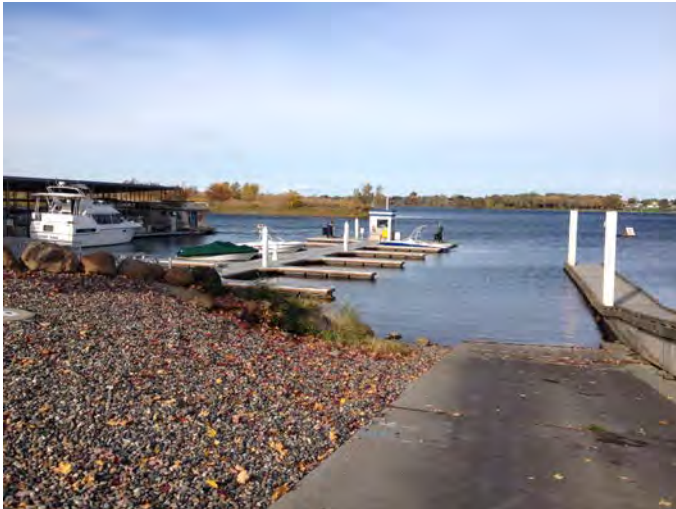
M-334.0R Photo: View of Columbia Park boat launch, fuel pumps, and location of Bateman Island where 2nd boom is to be anchored
