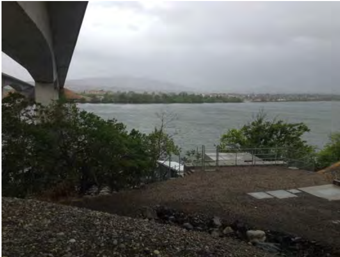
M-336.1-N Photo: Pasco Water Intake Facilities
