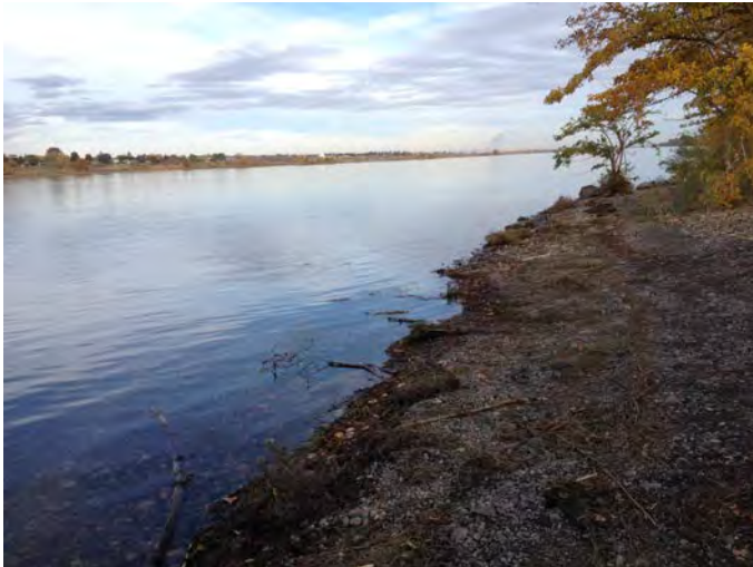
M-340.7L Photo: Looking upstream from Selph Landing toward where collection boom is to be placed
