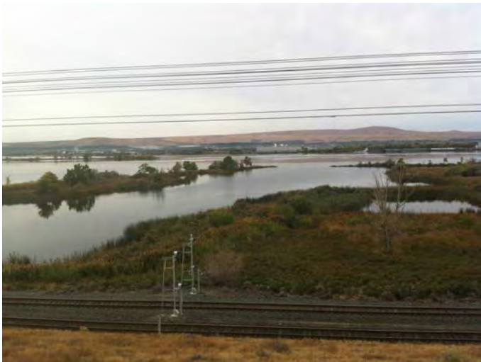
M-323.1M Photo: Boom off opening to prevent oil from reaching inner pond.
