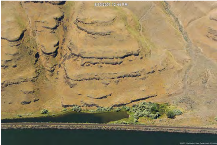
M-310.3R Photo: Aerial view of Switch Pond
