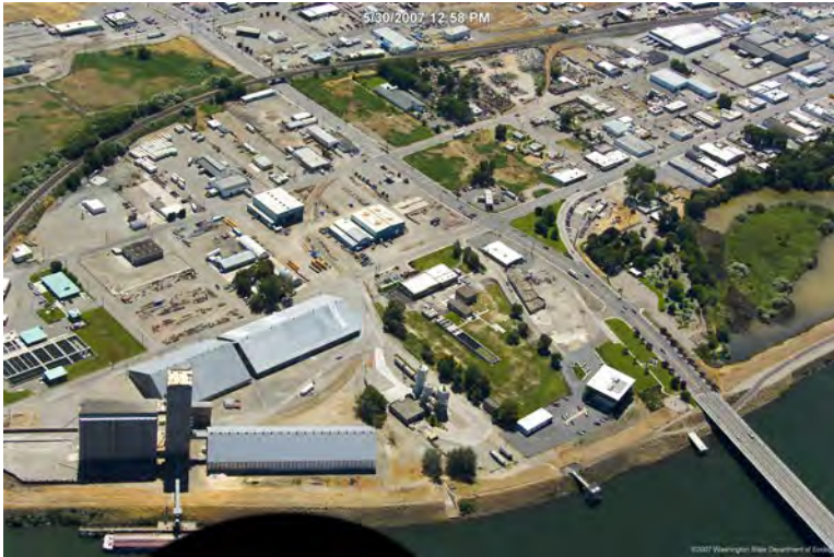
M-328.4-N Photo: Aerial view of the Kennewick Water Treatment Plant's water intake
