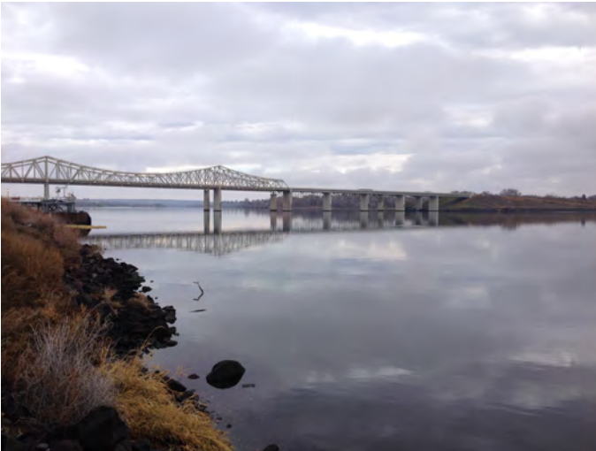
MSN-2.0R Photo: View from the Tesoro dock toward the bridge
