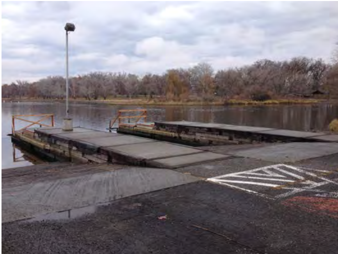
SA-MSN-2.3L Photo: Hood Park USACE boat launch
