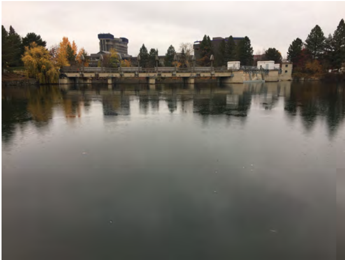
SPR-74.5-N Photo: From the Centennial Trail on Spokane River left, looking across the river towards Upper Falls Dam.
