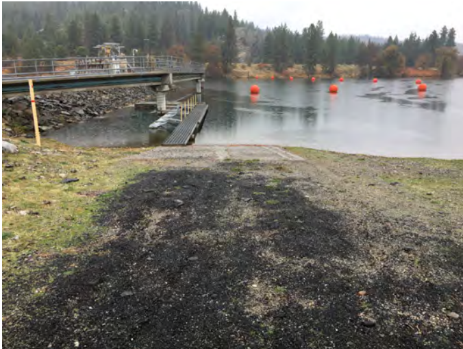
SA-SPR-80.0M Photo: From top of boat ramp on Spokane River right channel-left, looking at boat dock and cable barrier with Upriver Dam in background.
