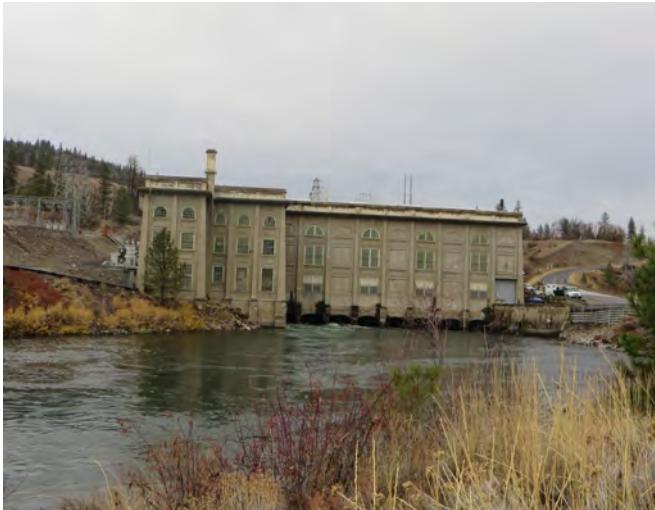
SPR-29.0-N Photo: From Little Falls Road on Spokane River left, looking upstream towards Little Falls Dam.
