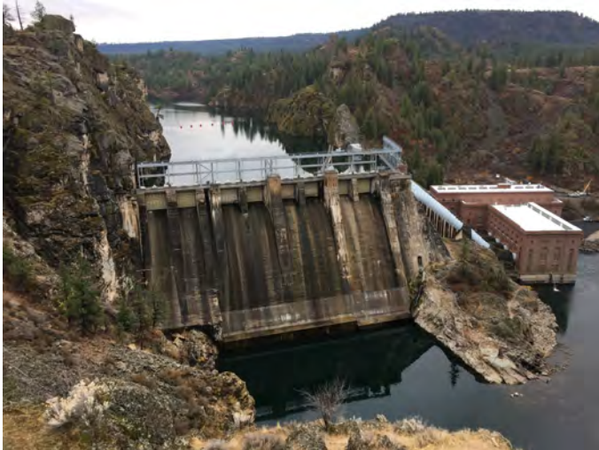
SPR-34.0-N Photo: From Highway 291 on Spokane River right, looking upstream towards Long Lake Dam.
