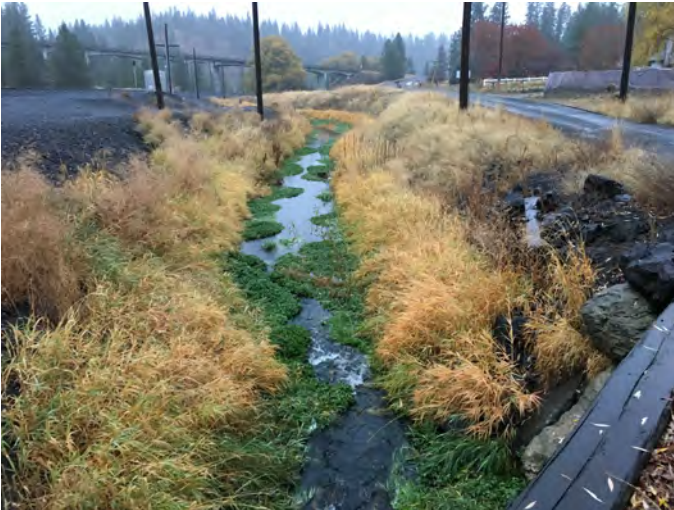
MHC-5.0R Photo: From bridge over Marshall Creek, looking downstream towards S Cheney-Spokane Road bridge.
