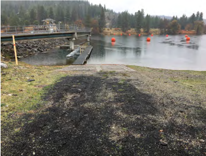
SA-SPR-80.0M Photo: From top of boat ramp on Spokane River right channel-left, looking at boat dock and cable barrier with Upriver Dam in background.
