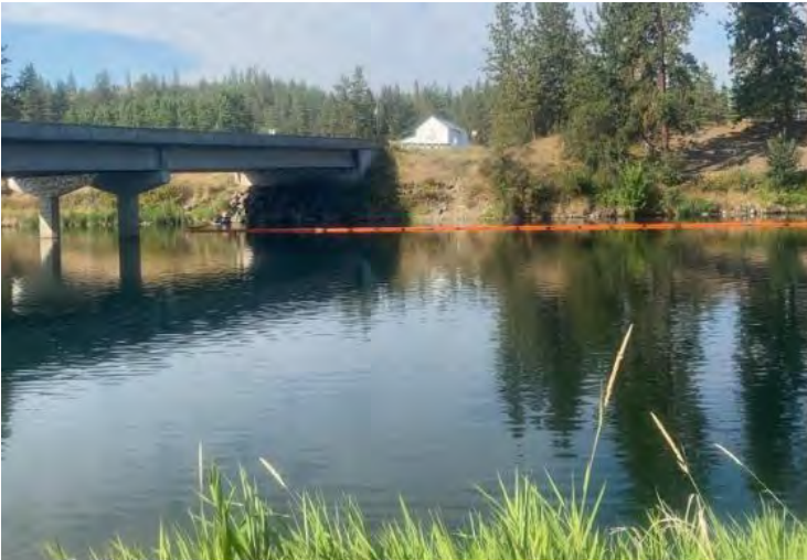
SPR-61.8R Photo: From right bank, looking southwest towards anchor point under the W 7 Mile Rd bridge. Photo was taken during a drill in July 2021.
