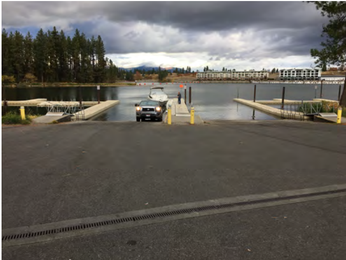
SA-SPR-102.5L Photo: From top of boat ramps on Spokane River left, looking across the river towards Post Falls Dam.
