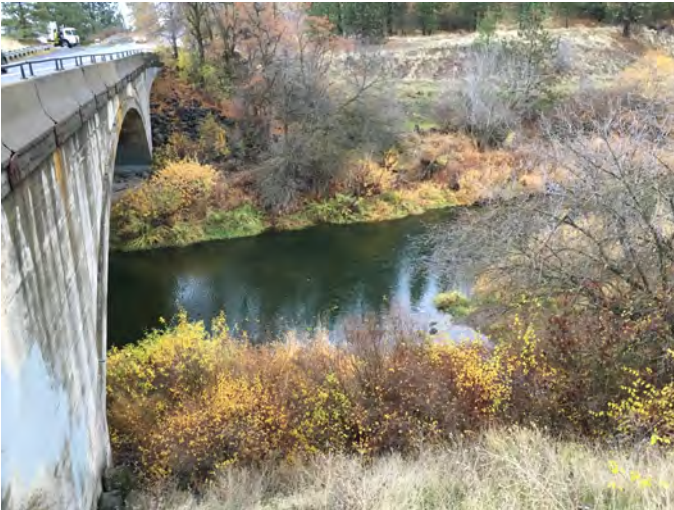
HMC-0.5R Photo: From southern end of Marne Bridge on Hangman Creek right, looking across the creek toward anchor point B.
