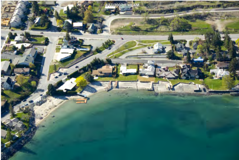
LKCH-61.0 Photo: Aerial photo looking south; strategy location is towards left side of photo
