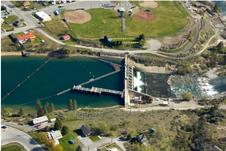
LKCH-60.2-N Photo: Aerial photo looking NE at Lake Chelan Dam
