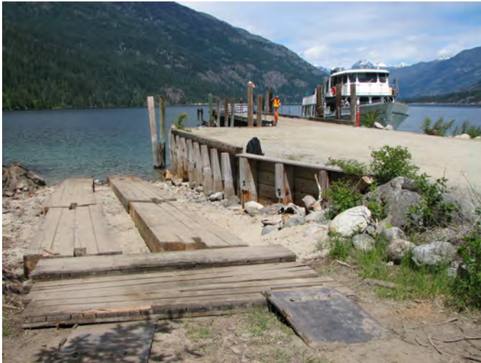
LKCH-108.5 Photo: Shoreside of SW corner of dock at Lucerne Landing, looking NW out towards Lake Chelan.
