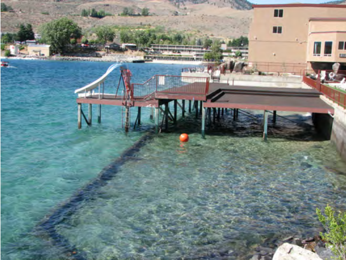
LKCH-60.8 Photo: From shore SW of strategy location, looking NE toward shoreside anchor point.
