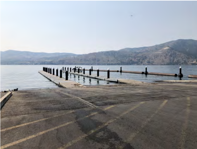
SA-LKCH-52.8 Photo: Looking South towards the boat launch
