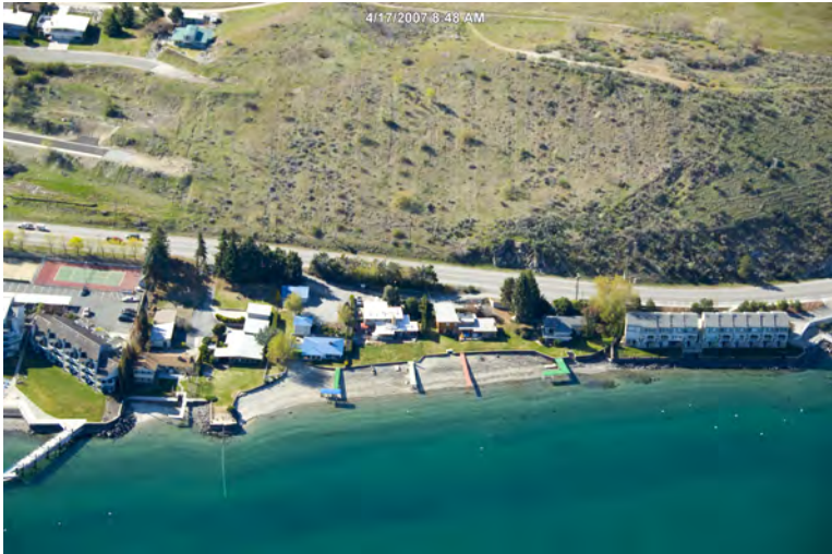
LKCH-61.2 Photo: Aerial photo looking south at strategy location; anchor point is dock on far left of photo.
