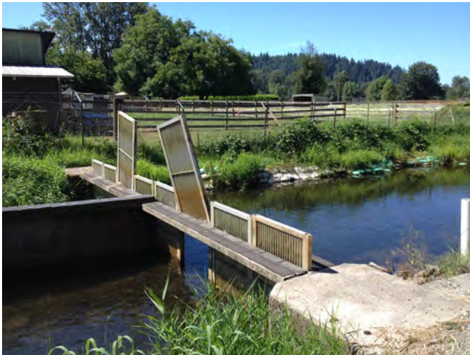
CRSP-1.2-N Photo: Fish gates on Crisp Creek to block fish coming/going to Green River.
