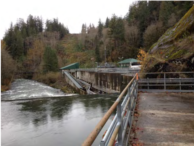
GRD-59.8-N Photo: Adult salmon ladder and water diversion dam for City of Tacoma water supply. Looking W downstream from water intake on river right.
