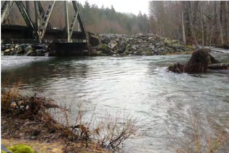
UGR-80.9 Photo: From river right, looking SW upstream at strategy location.
